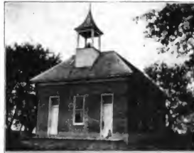
Rochester Schoolhouse After Rebuilding
